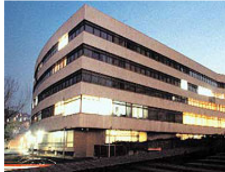
Joint Institutions' building, Sarajevo
